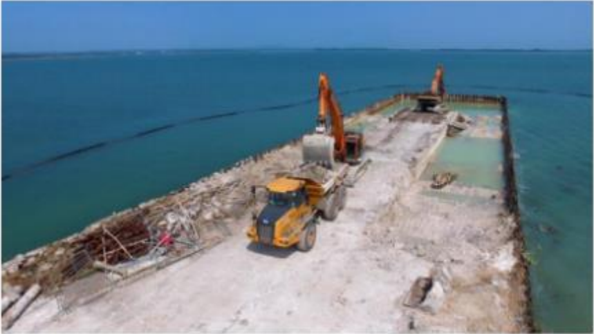
Chalk fill and sheet piles removed from quay ~2,500m 2 new mud flat created
