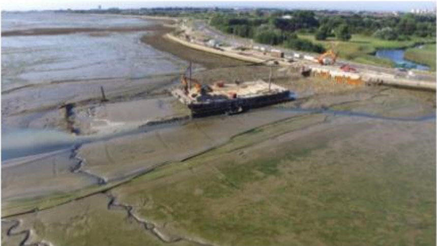
Chalk fill and sheet piles removed from quay ~2,500m 2 new mud flat created
