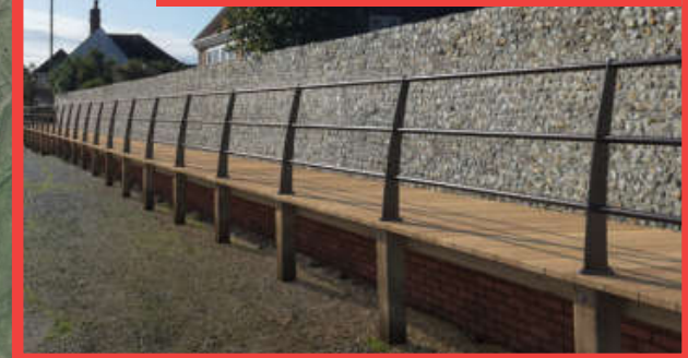
Floodwall with boardwalk
