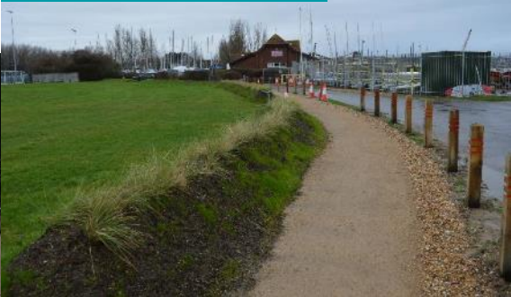
New paths installed
