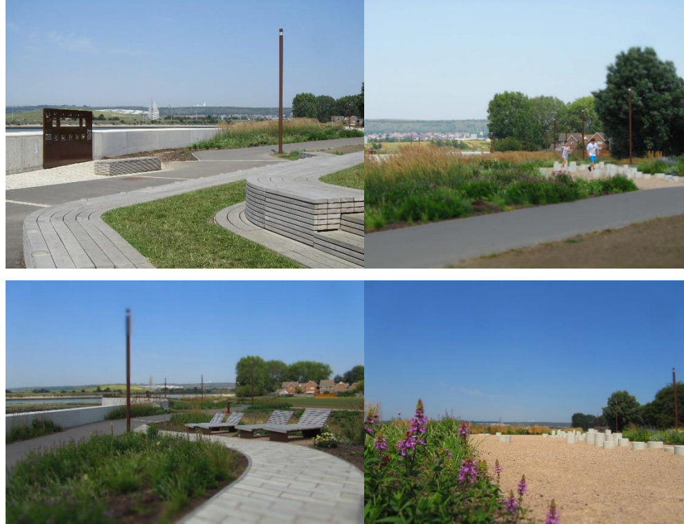
Tipner Coastal Defence Scheme post completion
