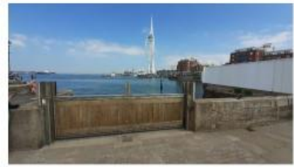
Point Slipway: Adding additional boards
