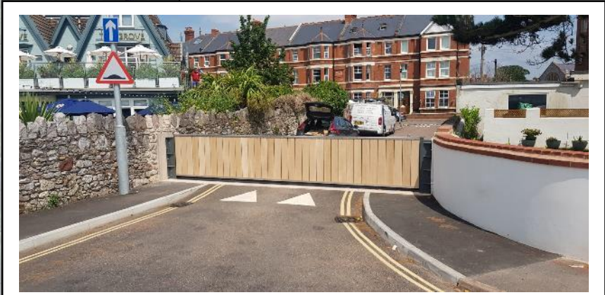
Timber Cladded Flood Gate – Exmouth Flood Control International
