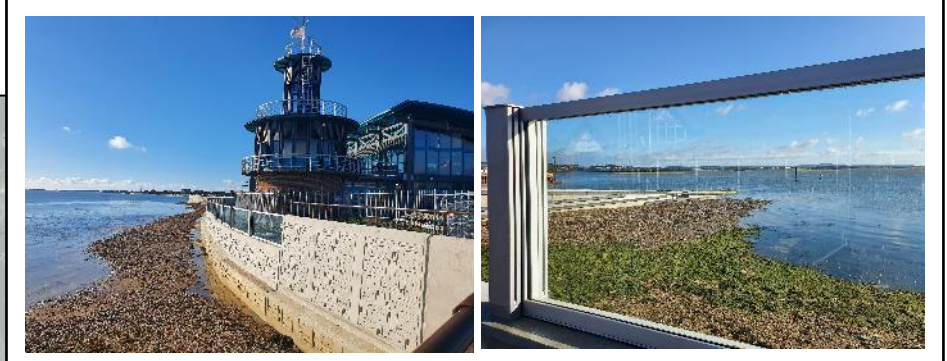
Glass Flood Barrier, North Portsea Island
