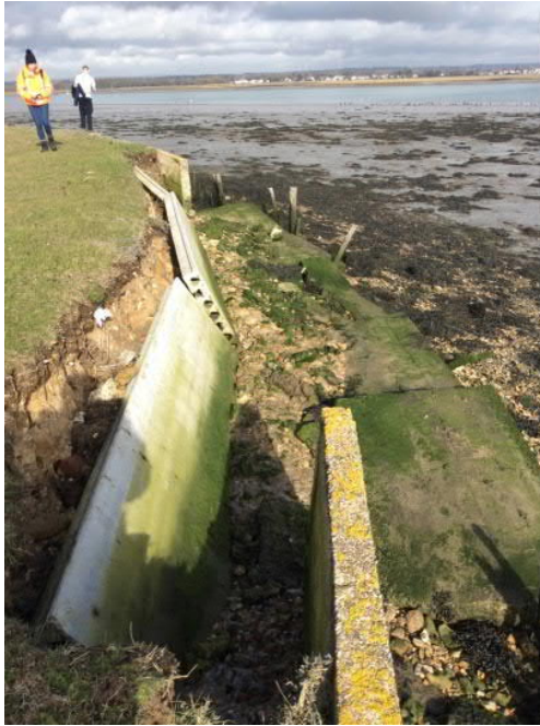
Figure 7-2. Photographs of failed defences between 5AH102 A-E
