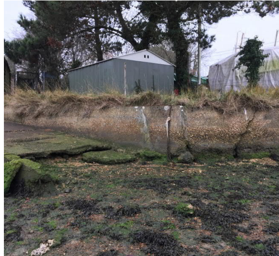
Figure 7-3. Photograph of 5AH104 section A showing lateral crack
