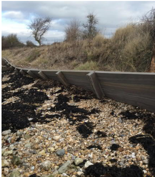
Figure 7-6. Timber defences in sections D and F
