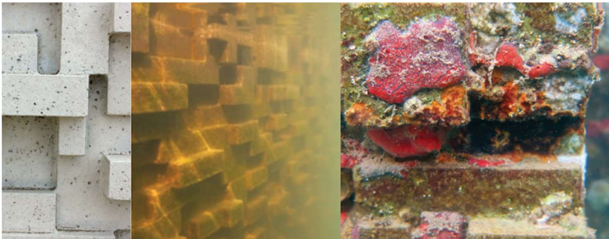
Figure 23-9 EConcrete modular seawall units 42 .
