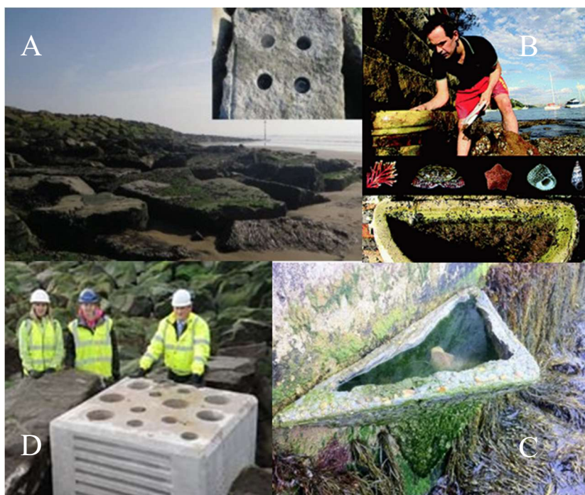
Figure 23-10 (A) Drilled rock pools, (B) Flower pot rock pools, (C) Vertipool, (D) BIOBLOCK rock pools 43 .
