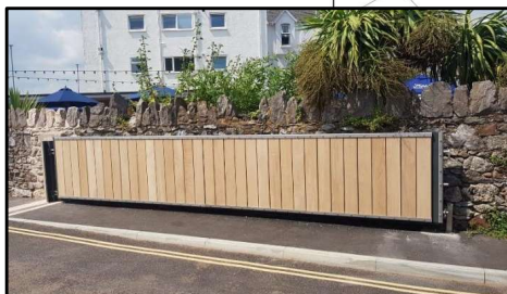
Timber Cladded Flood Gates
