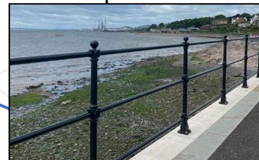
Handrails – (Whole Length)
