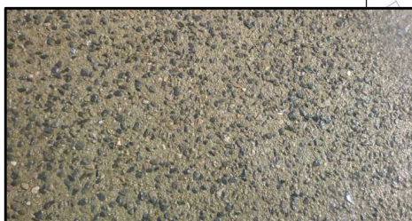
Exposed Aggregate Footpath (Whole Length)
