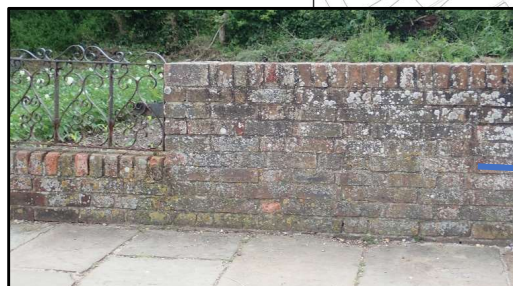
Existing Brick Wall Retained
