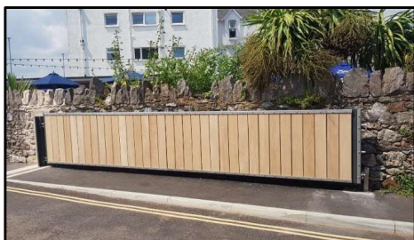
Timber Cladded Vehicle Flood Gates
