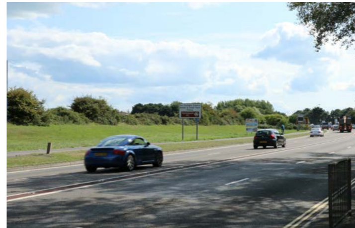
Photo 17 Looking south east along Eastern Road
