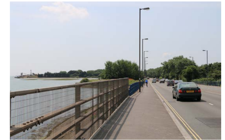
Photo 20 looking south on Eastern Road Bridge
