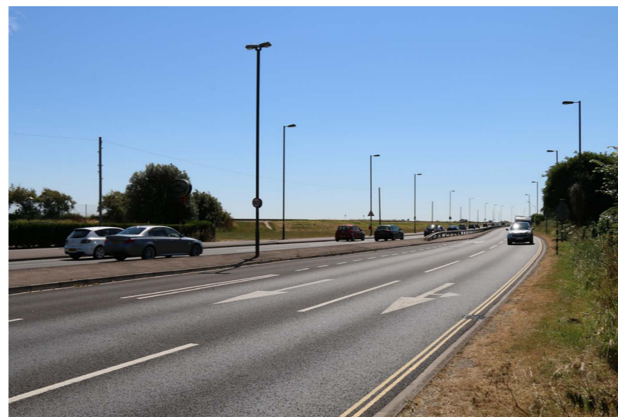
Photo 20 Looking south east from the footpath adjacent the petrol station on Eastern Road. The coast path is considerably higher than the road level at this point, preventing views to the harbour from the road
