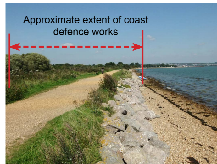
Photo 11 View of Coast Path looking north, with recent rock revetment. New works will be similar in character and scope to this
