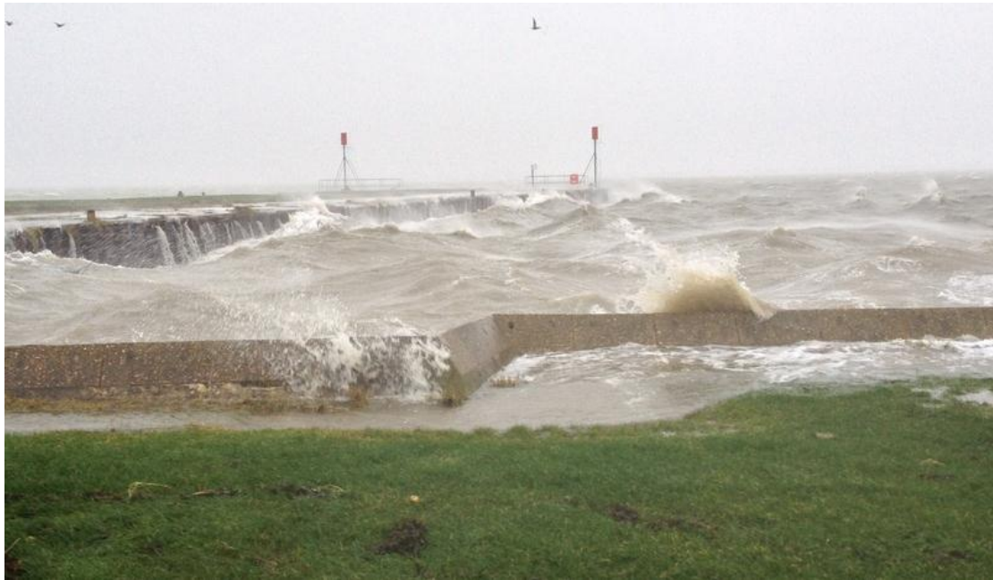
Plate 6.3 Flooding of the Eastern Road caused by wave overtopping at Great Salterns Quay (3 rd January 2014):
