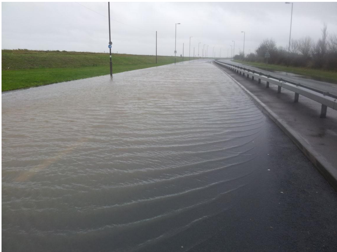
Plate 6.3 Flooding of the Eastern Road caused by wave overtopping at Great Salterns Quay (3 rd January 2014):
