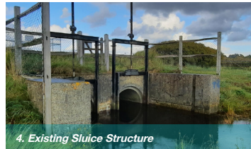
4. Existing Sluice Structure
