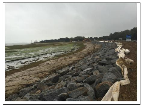
Photo 3.3: Typical rock revetment structure between Eastern Road Bridge and Kendalls Wharf
