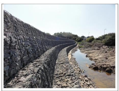
Photo 3.4: Typical view of gabion retaining wall adjacent to the Eastern Road Balancing Pond
