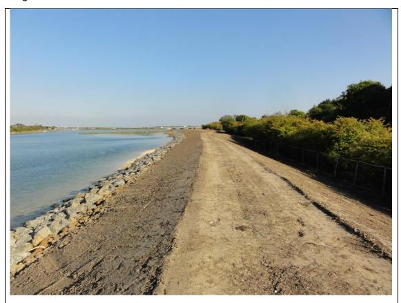
Photo 5.3: Newly constructed flood banks and revetment along Ports Creek. Note the limited footprint of impact, following tight control measures.
