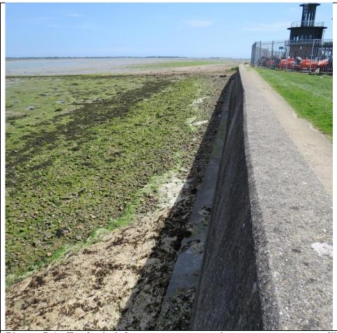
Photo 5.1: Typical defence structure where encasement will occur, causing encroachment of 400mm onto the foreshore (into the shaded area). This section of seawall is within Langstone Harbour, to the northern end of the Eastern Road frontage.
