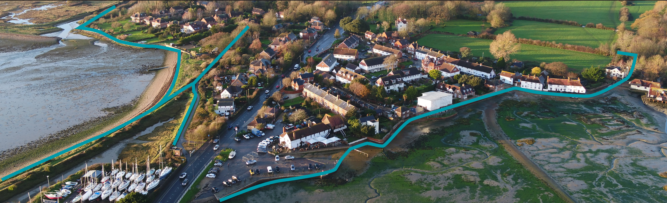
Aerial image annotated to show extent of GI works
