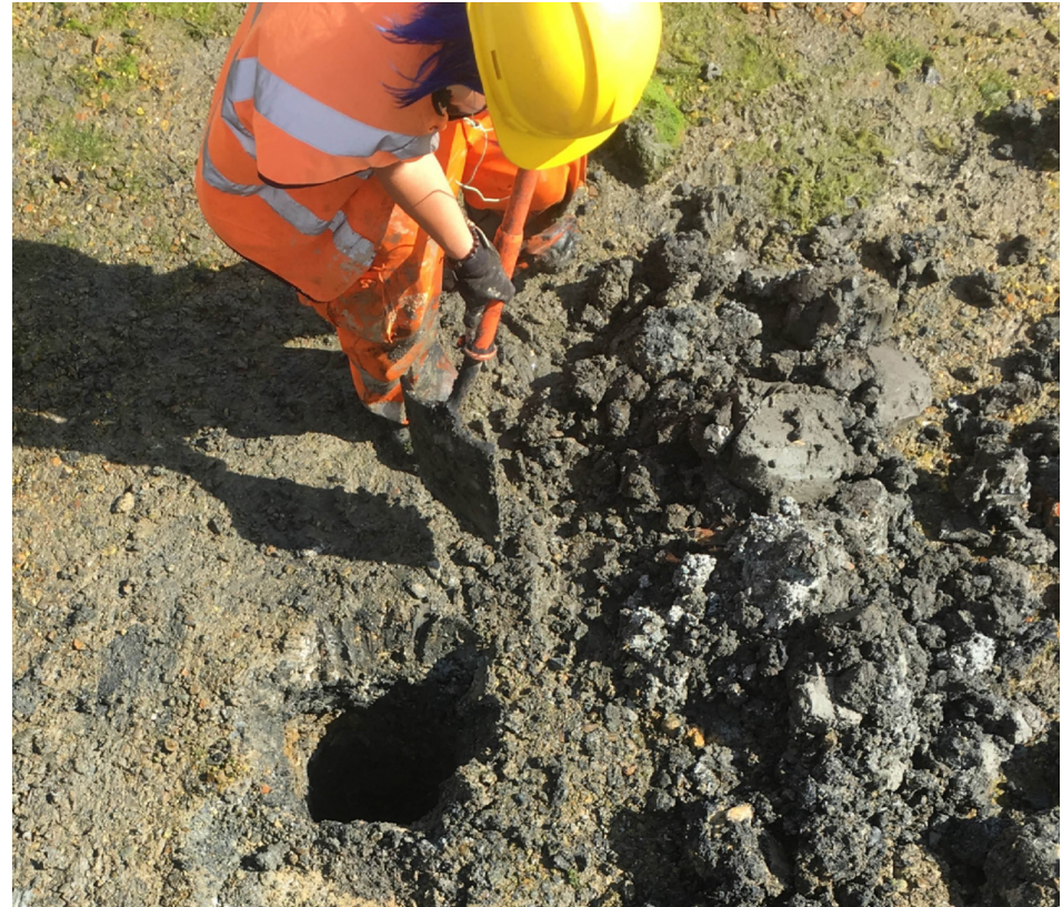
Trial pit undertaken at Langstone in September 2018
