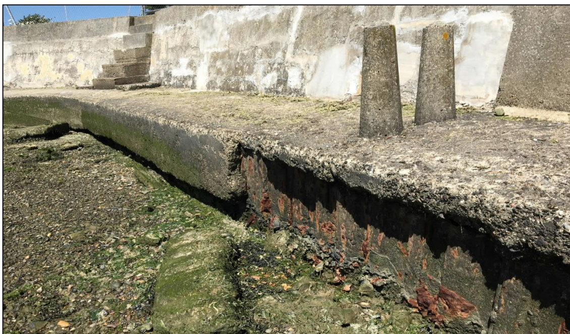
Figure 4-3: Existing seawall in ODU 1b
