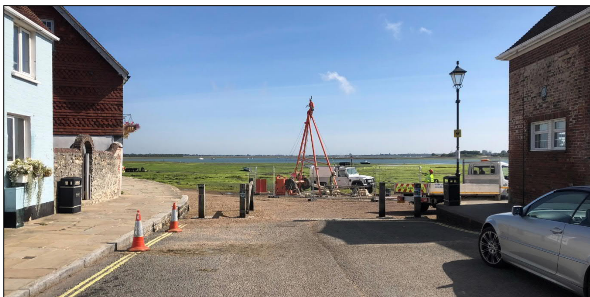
Figure 4-18: Photograph of Langstone High Street slipway
