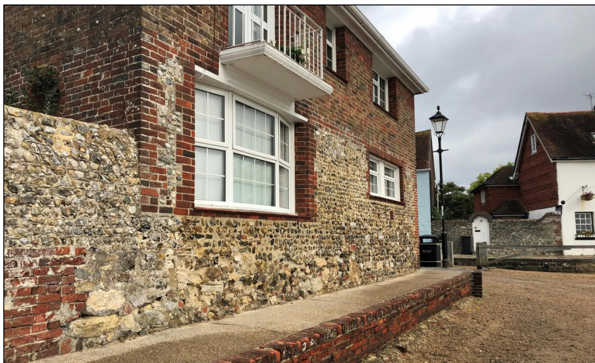
Figure 4-17: Photograph of residential building and footpath in ODU 3i
