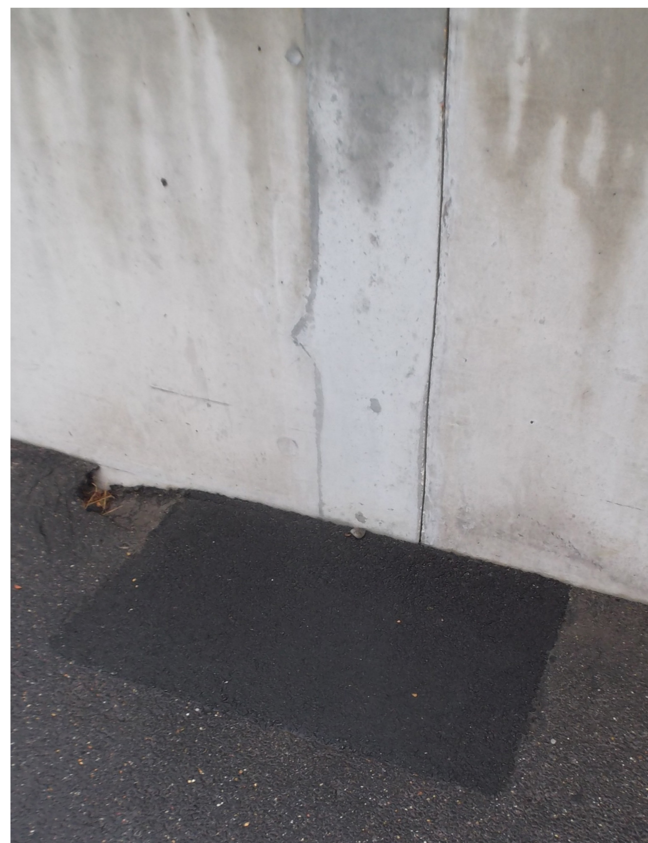
5. Removing shutters and replacing tarmac surface.
