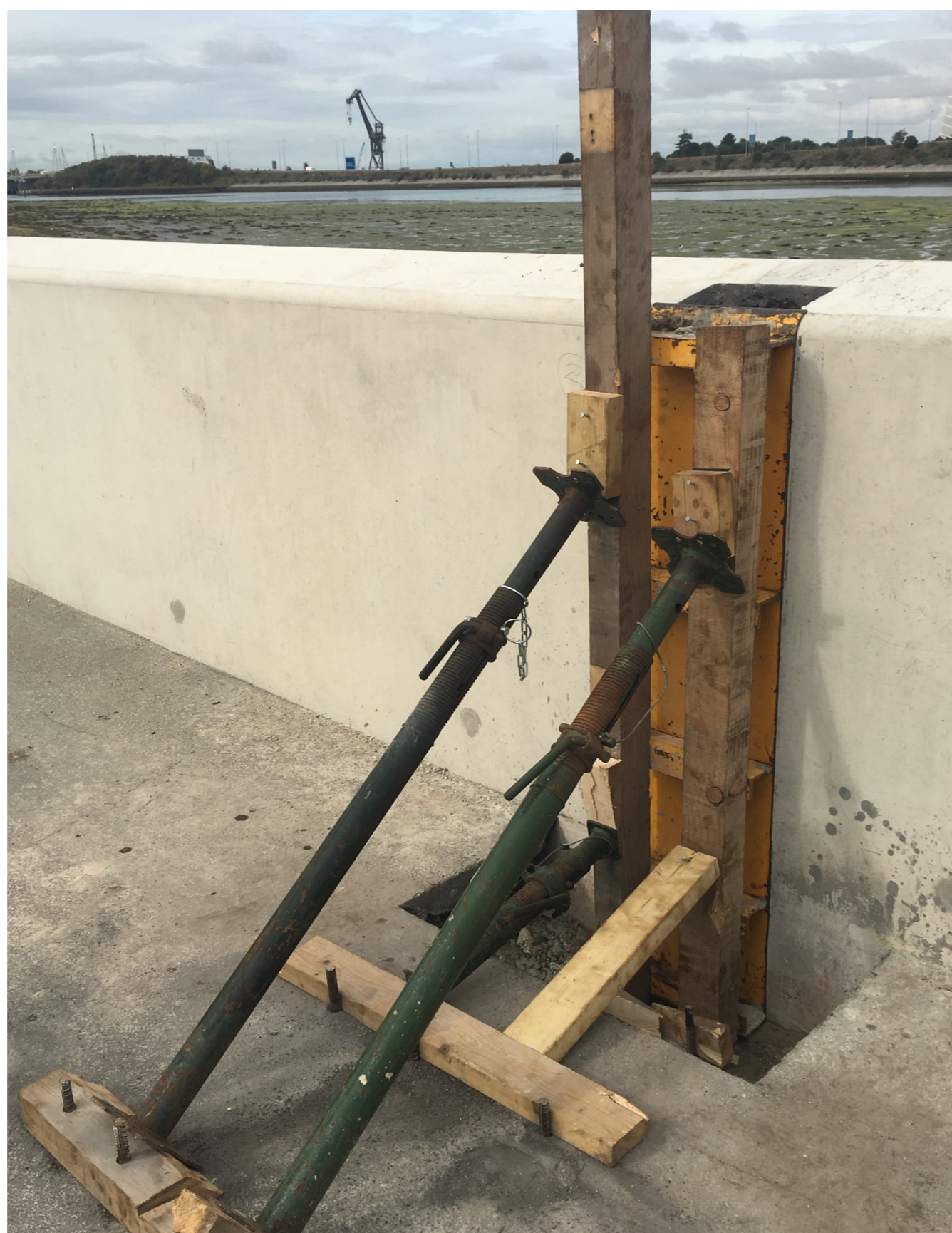
4. Attaching shutters and pouring concrete
