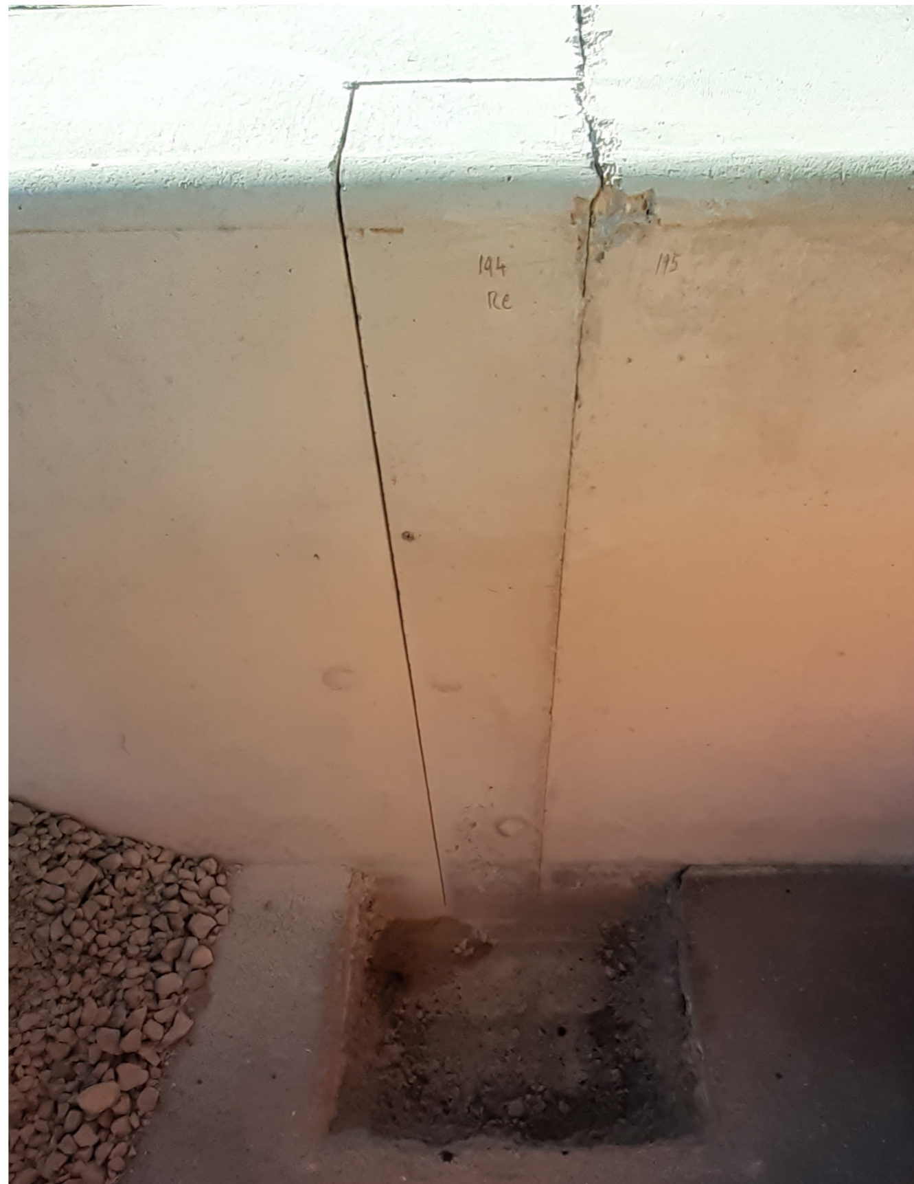
2. Cutting the area of wall with a saw, ready for removal
