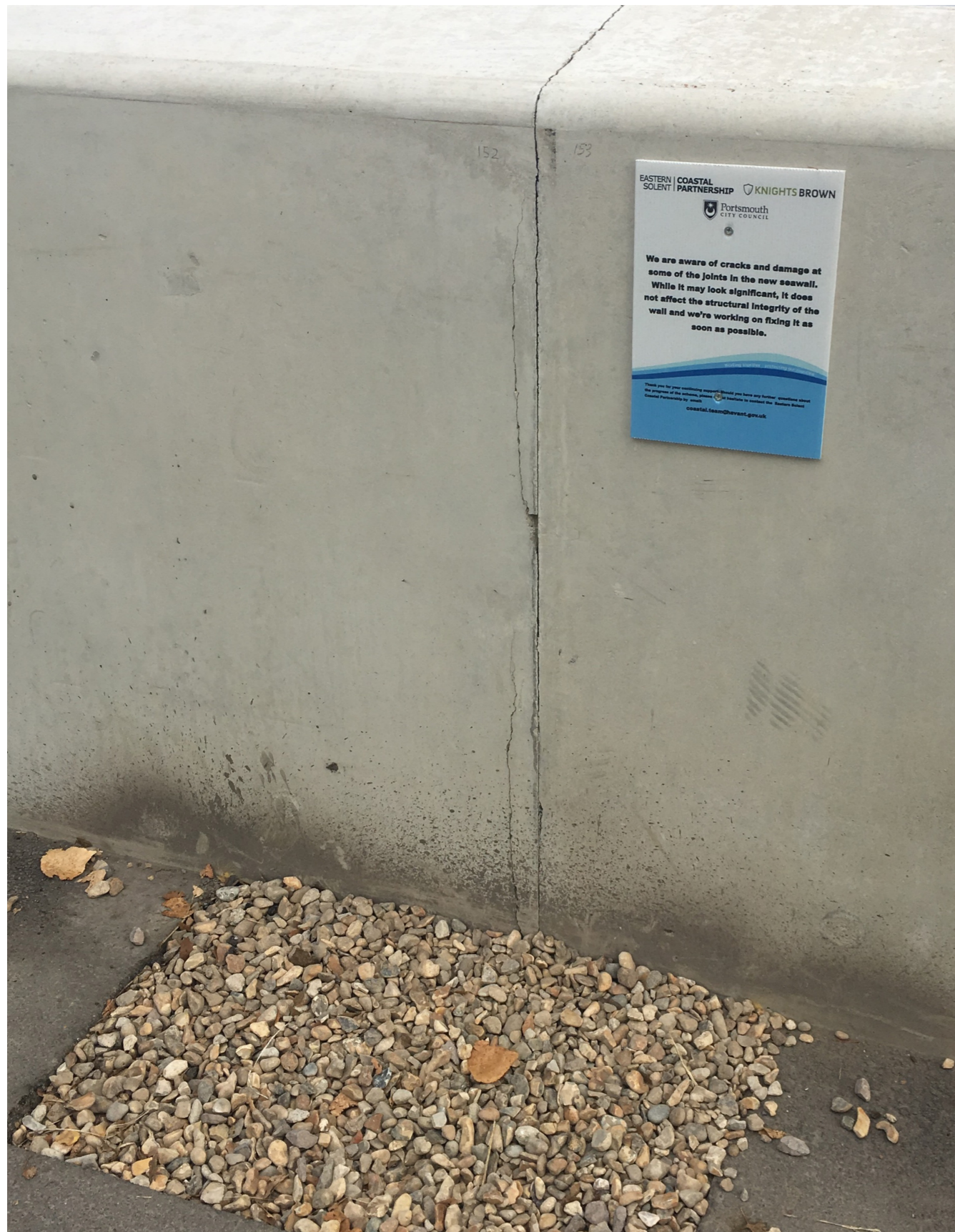
1. Removing tarmac and ground to expose wall joint
