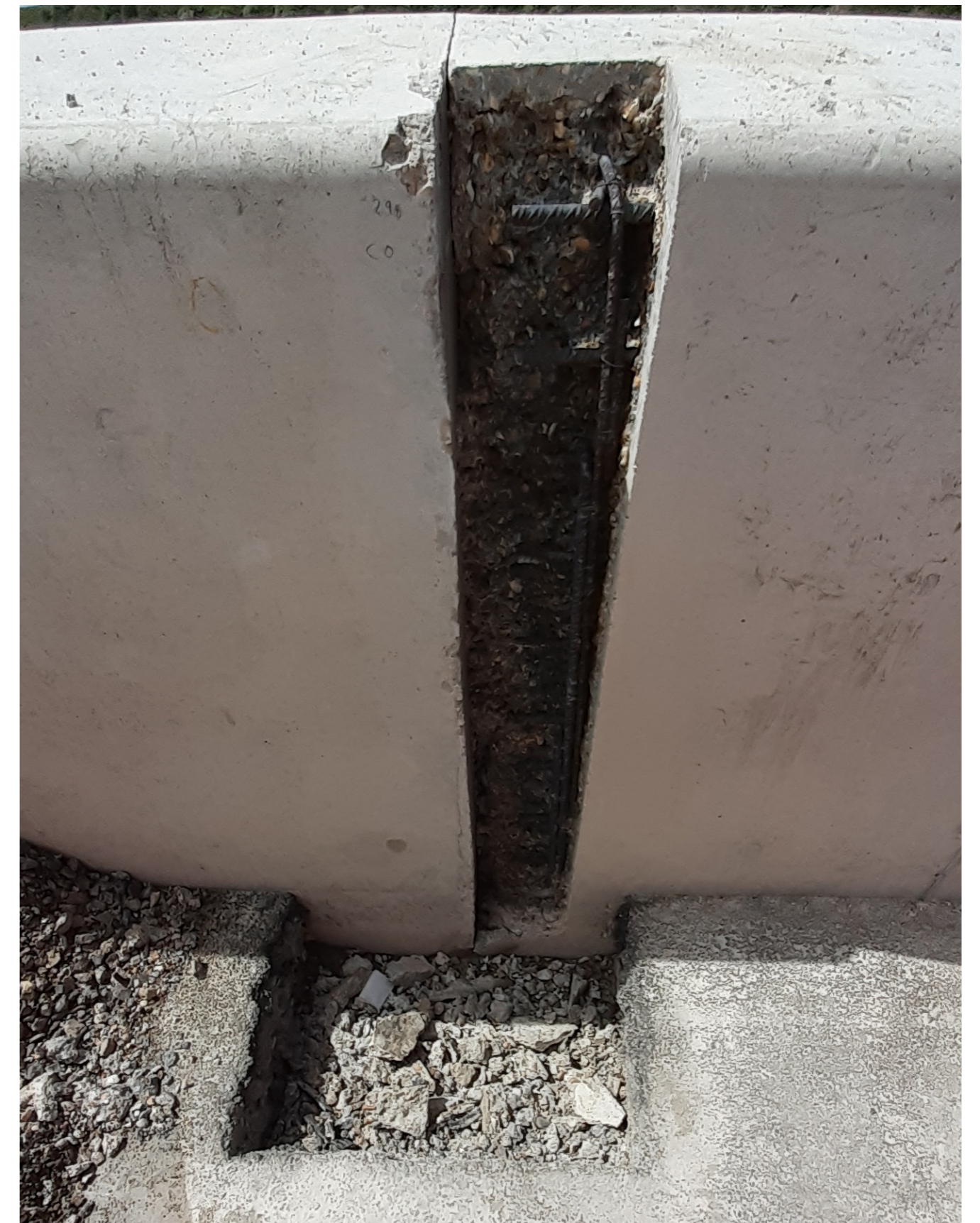
3. Removing concrete using 'hydro-demolition' (a strong jet of water) and removing small rubber strip
