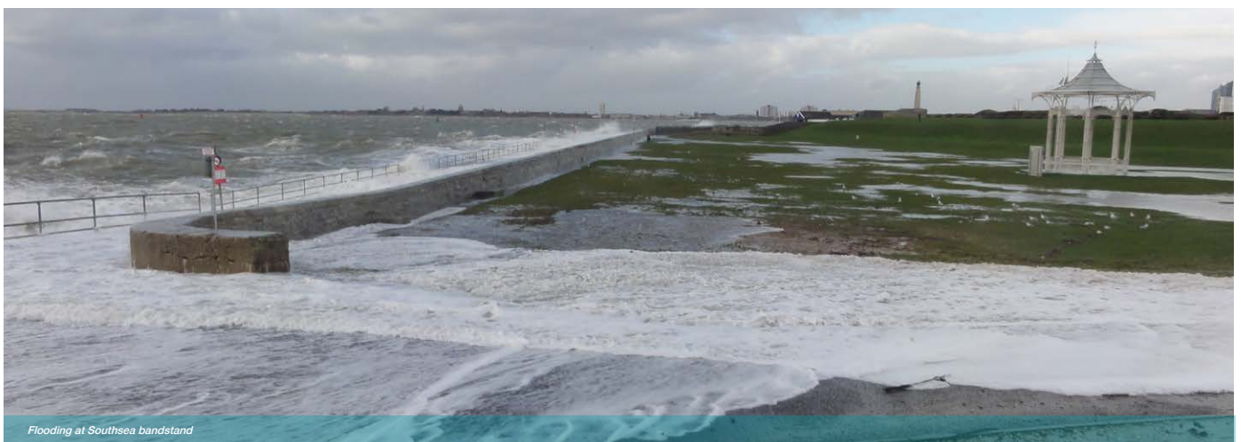
Flooding at Southsea bandstand
