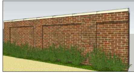
BRICK CLAD FLOOD WALL WITH RECESSED PANELS AND STONE COPING
