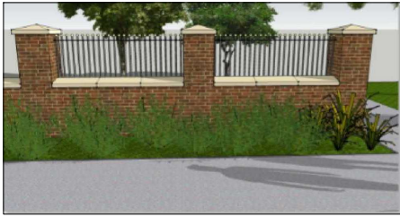
BRICK CLAD FLOOD WALL WITH PIERS, STONE COPINGS AND INFILL RAILING PANELS
