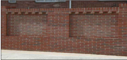
RECESSED BRICK CLADDING
