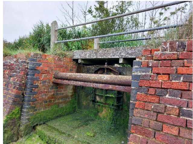
Figure 16 (Left) outfall/weir from the mill pond; (Right) sluice controlling fresh and brackish water outlet/inlet (Photographs taken during site visit 9 th August 2023)
