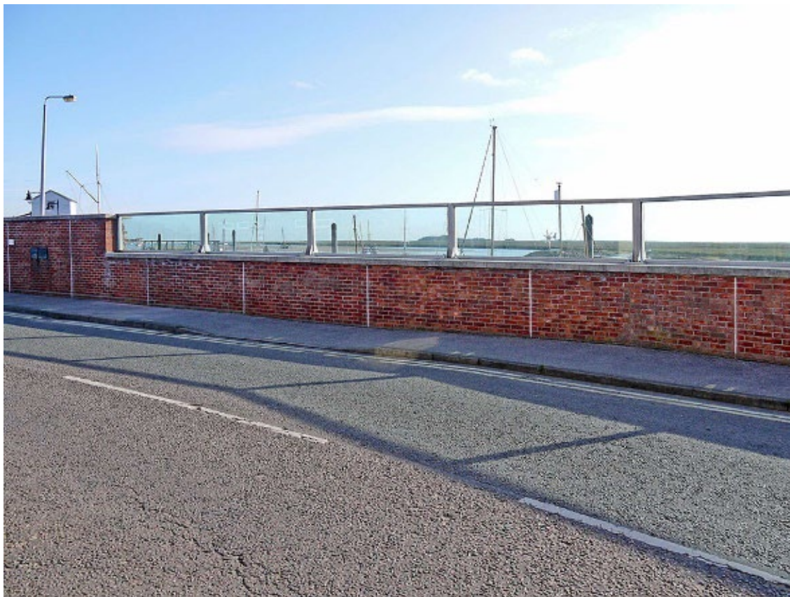
Figure 29: Example of glass and masonry seawall in Wells on the sea, Norfolk.
