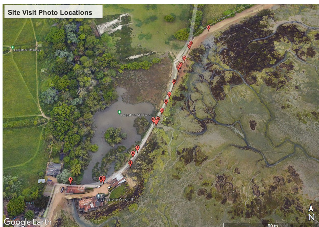
Figure 5 Representative locations of photos taken during the inspection.
