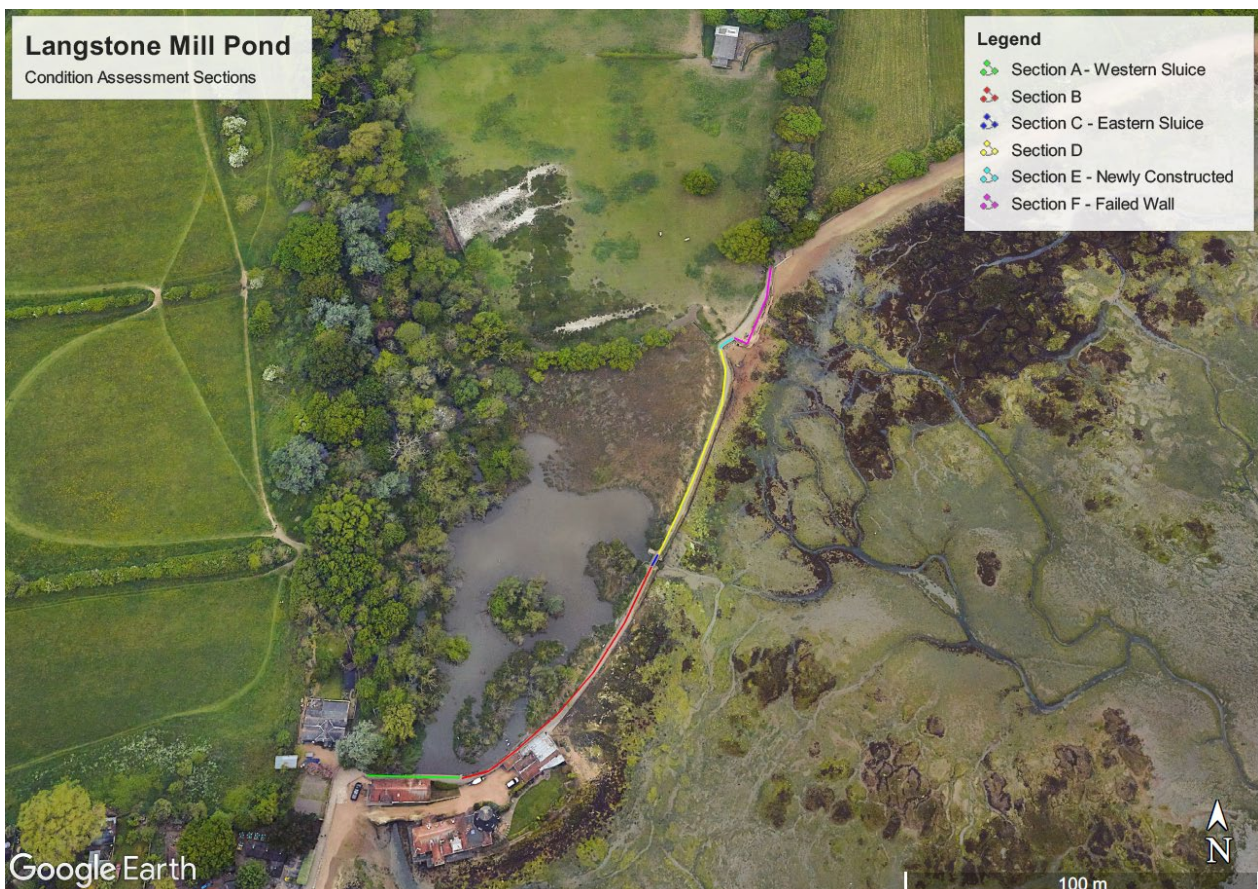
Figure 2: Overview of the coastal defences around Langstone Mill, including condition assessment sections.
