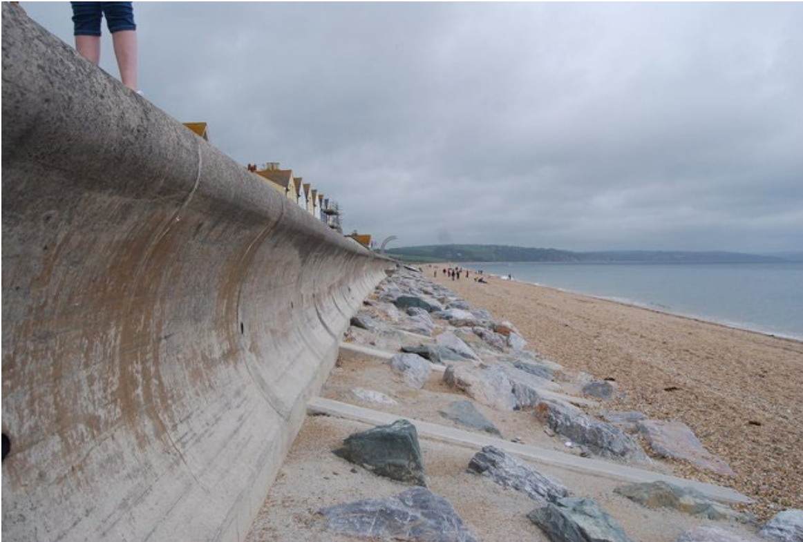
Figure 28: Example of a concrete seawall at Torcross, Devon, where the path is on top of the seawall crest.
