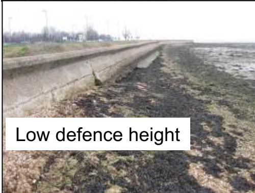
Tidal flooding A2030- Eastern Road Jan 2014
