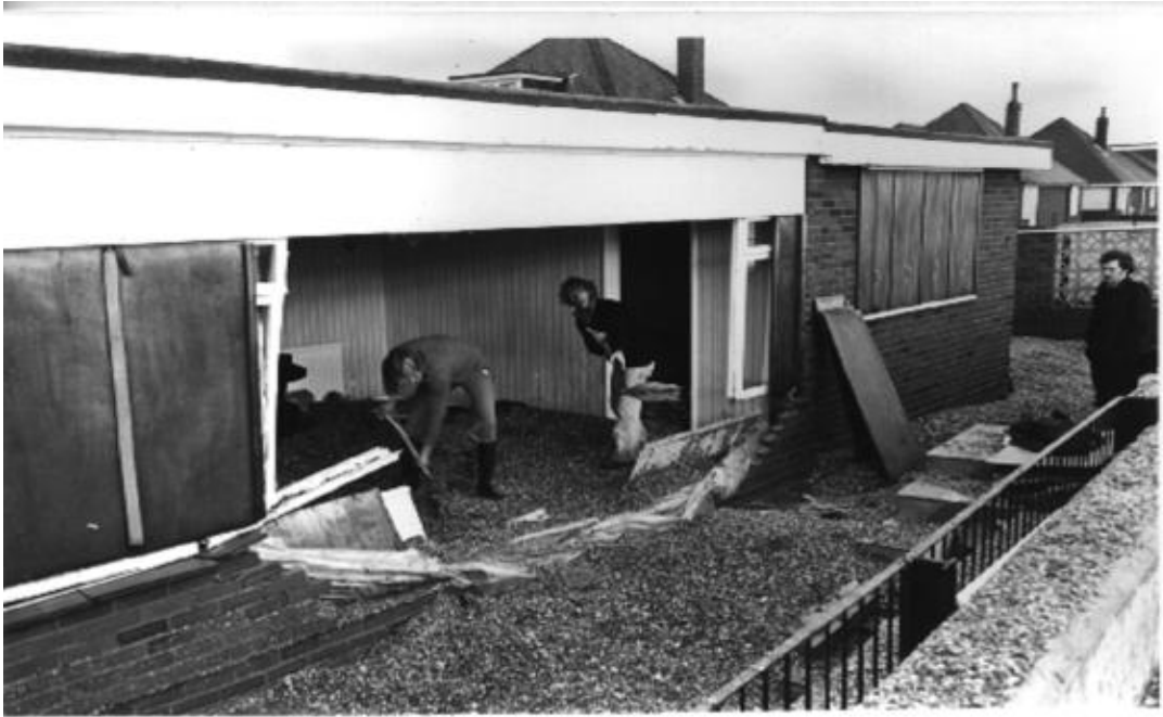
Plate 1.1 - Storm damage to property behind the promenade, December 1978.
