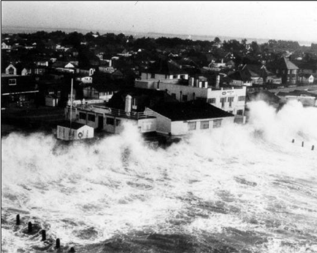
Plate 1.3 - Wave overtopping adjacent to Creek Road car park, Pre-Beach Replenishment 1985
