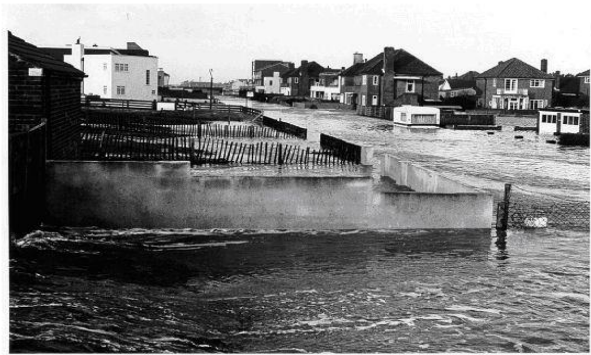
Plate 1.2 - Storm damage to properties behind the seawall, December 1978.
