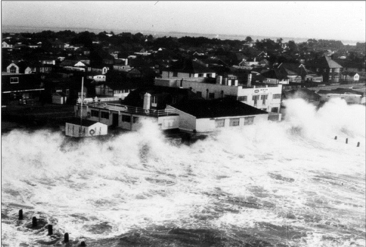
Plate 1.3 Wave overtopping adjacent to Creek Road car park, pre Beach Replenishment 1985
